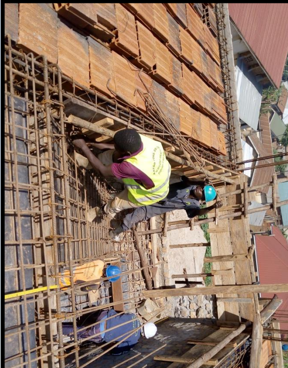
Steel works for staircases at Midland High School Kawempe site
